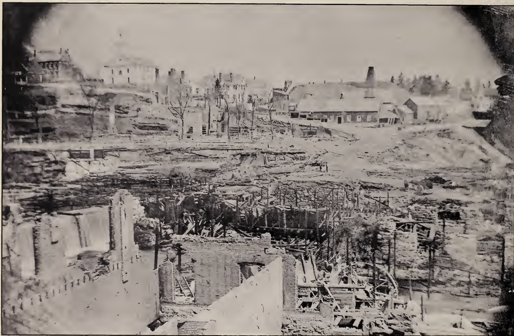
AFTER THE FIRE, APRIL 25, 1860.
